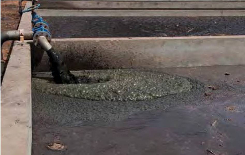
Figure 7.4 Loading of the beds at Niayes faecal sludge treatment plant, Dakar, Senegal (photo: Linda Strande).
