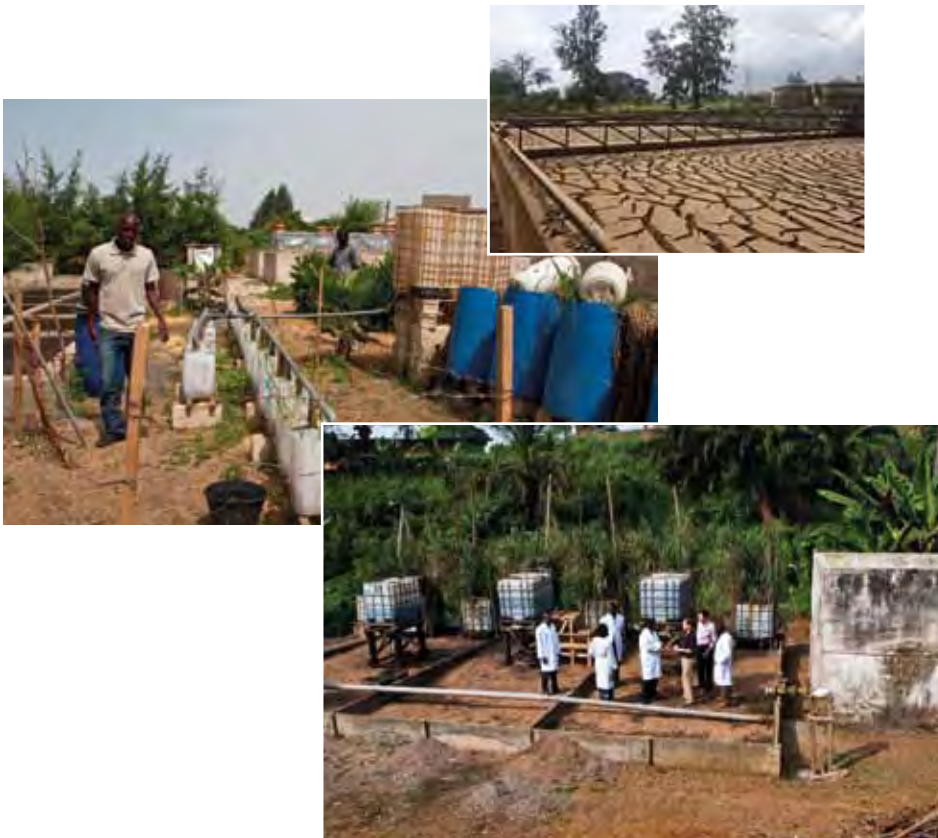
Figure 18.5 Drying bed research: mixing device for unplanted faecal sludge drying beds at Bugolobi wastewater treatment plant in Kampala, Uganda; evaluating potential plant species for planted drying beds in Dakar, Senegal; and planted drying bed pilot for treatment of drying bed leachate in Yaoundé, Cameroon (photo: Linda Strande).
