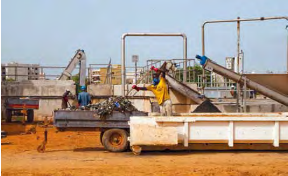
Figure 11.1 Maintenance worker cleans mechanical screens, a critical activity to be performed each shift to keep the system operational, Dakar, Senegal (photo: Linda Strande).
