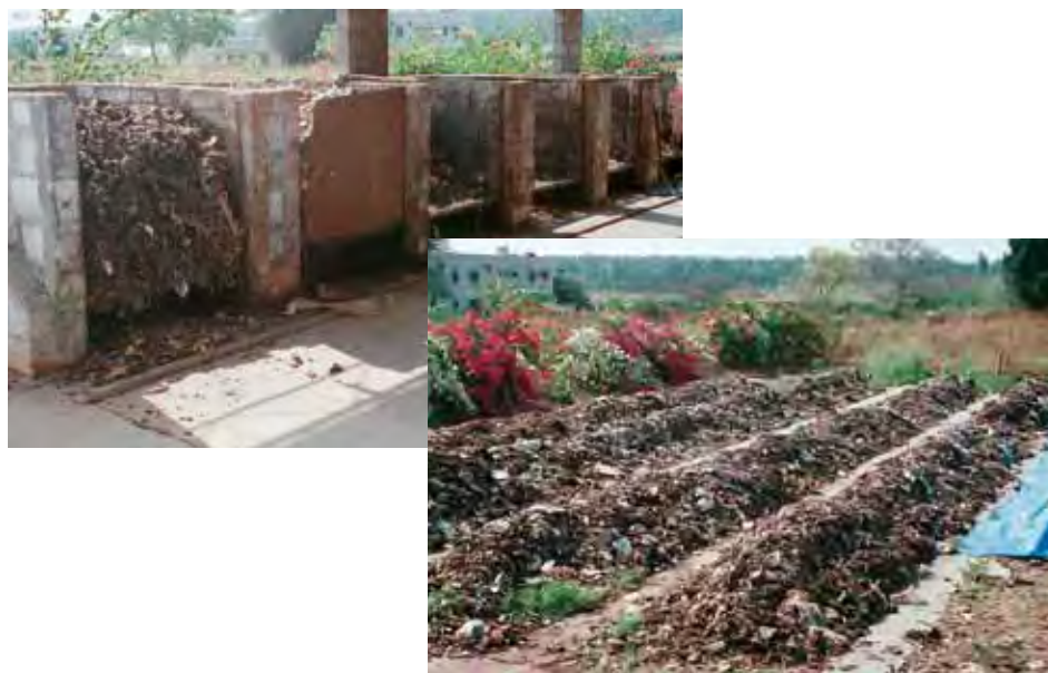
Figure 3.11 Pilot scale co-composting facility with faecal sludge and municipal waste in Bangalore, India (photo: Chris Zurbrugg).
