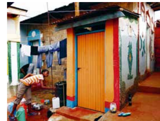
Ubsup toilet facility, Kenya
