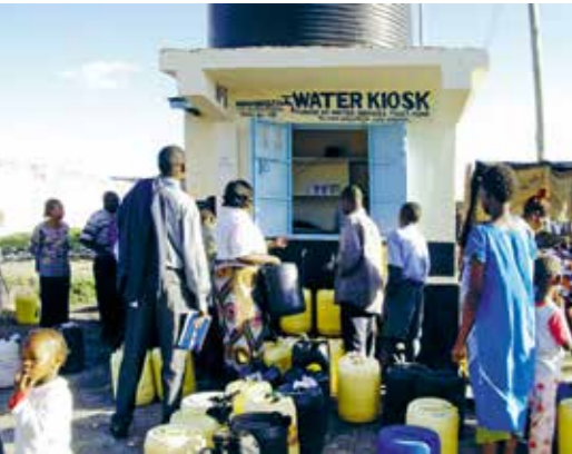
Utility operated water kiosk, Kenya
