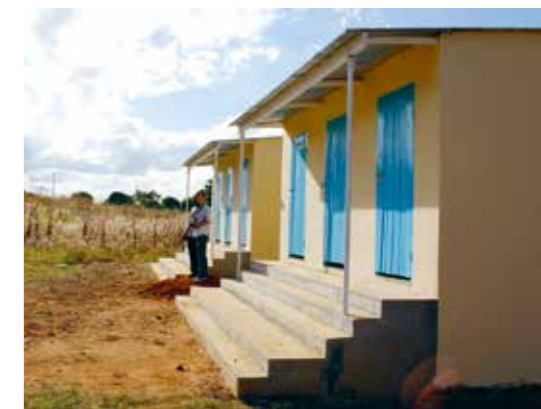
School sanitation facility, Zambia
